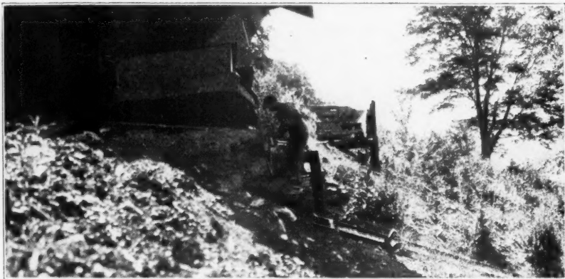
Dump Car on Incline About to Descend from the End of Railroad to the Mill.
